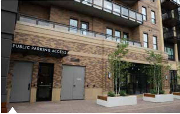
The Center Ramp was completed as a part of Nolan Mains at 50th & France last fall. Photo by Kaylin Eidsness
