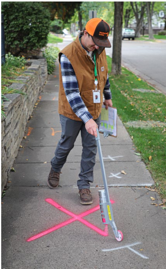
Derek Leonard marks a sidewalk panel for replacement in the Country Club Neighborhood. (Photo by Brittany Bader)
