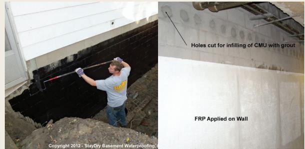
(Left) Example of exterior application of asphalt membrane (courtesy of <https://staydrywaterproofing.com/>) (Right) An interior application of a fiber-reinforced polymer wrap, image provided by FEMA P-312, Homeowner's Guide to Retrofitting 3rd Edition (2014)
