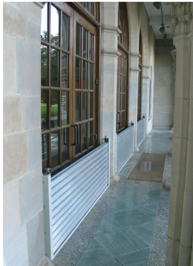
(Above) Metal shields installed with bolts or permanently installed tracks; image courtesy of [www.psfloodbarriers.com/wp-content/uploads/sites/4/2016/09/Flood-Plank-21.jpg](http://www.psfloodbarriers.com/wp-content/uploads/sites/4/2016/09/Flood-Plank-21.jpg)
